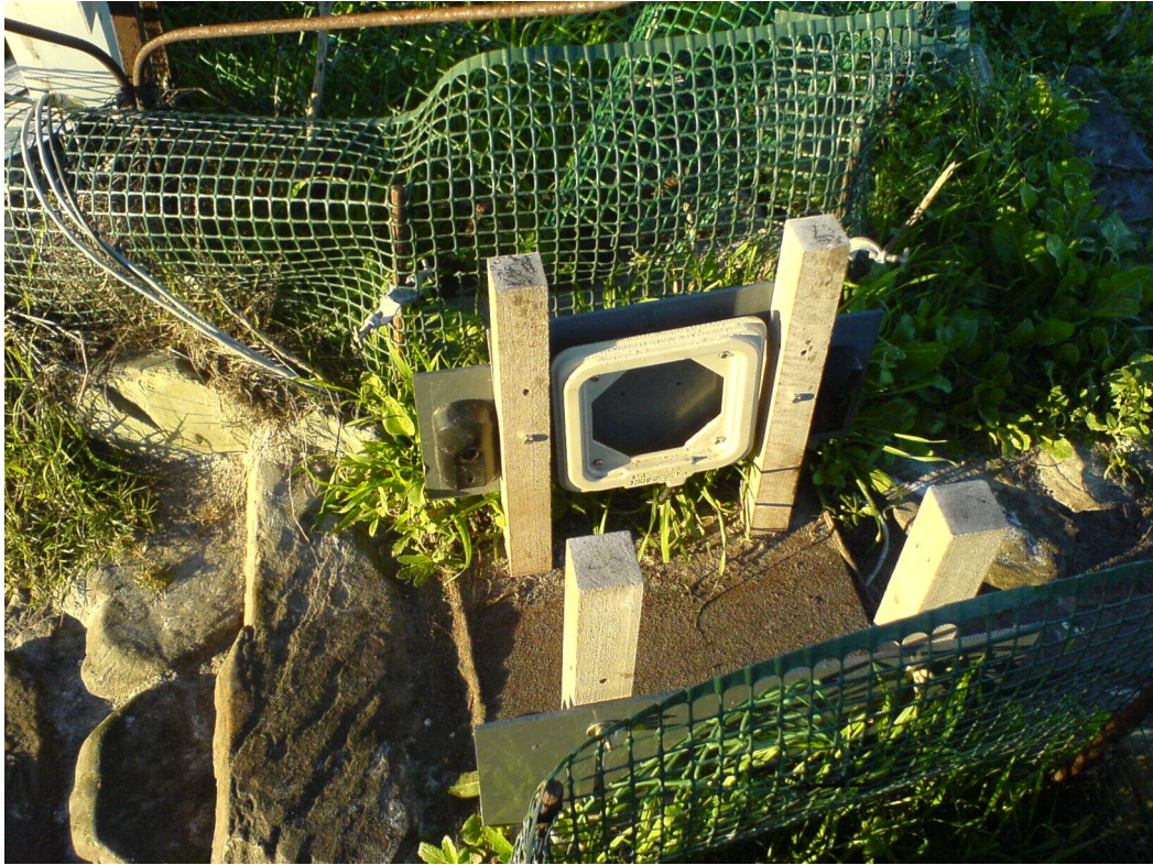
Figure 2.2: Existing system: close-up of the gate showing the Texas Instruments Series 2000 “small” loop antenna and the two infra-red beam detectors.
