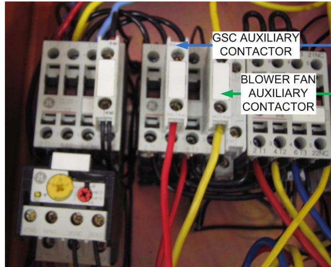
Figure 5.5: Re-wiring the blower fan starter via an auxiliary contact on the soft starter.
