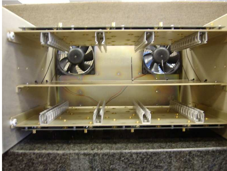
Figure 4.12: The 19" RF rack accommodates all the hardware of the 24-channel RF receiver. The top and bottom level are for the two motherboards, with the two synthesiser boards sandwiched in between them.
