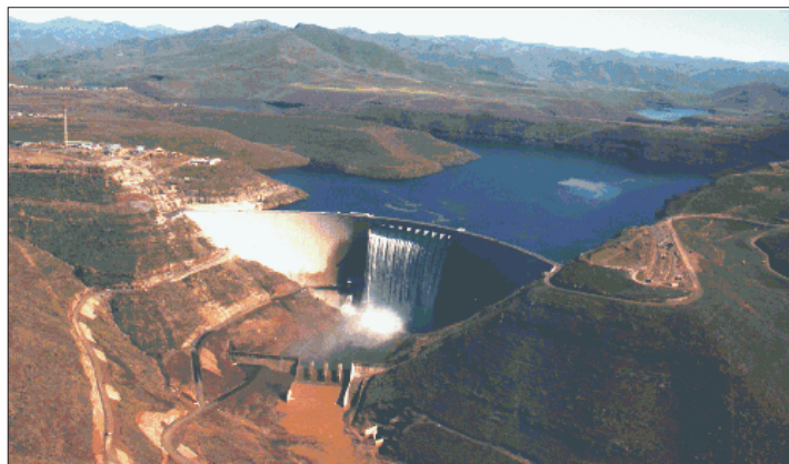
Figure 4.2: Katse Dam - Keystone of the Lesotho Highlands Water Project
