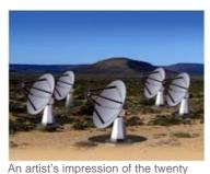
dishes of the Karoo Array Telescope on site near Carnarvon in the Northern Cape. Each of the 20 dishes will be 15 m in diameter and about 19 m high.
